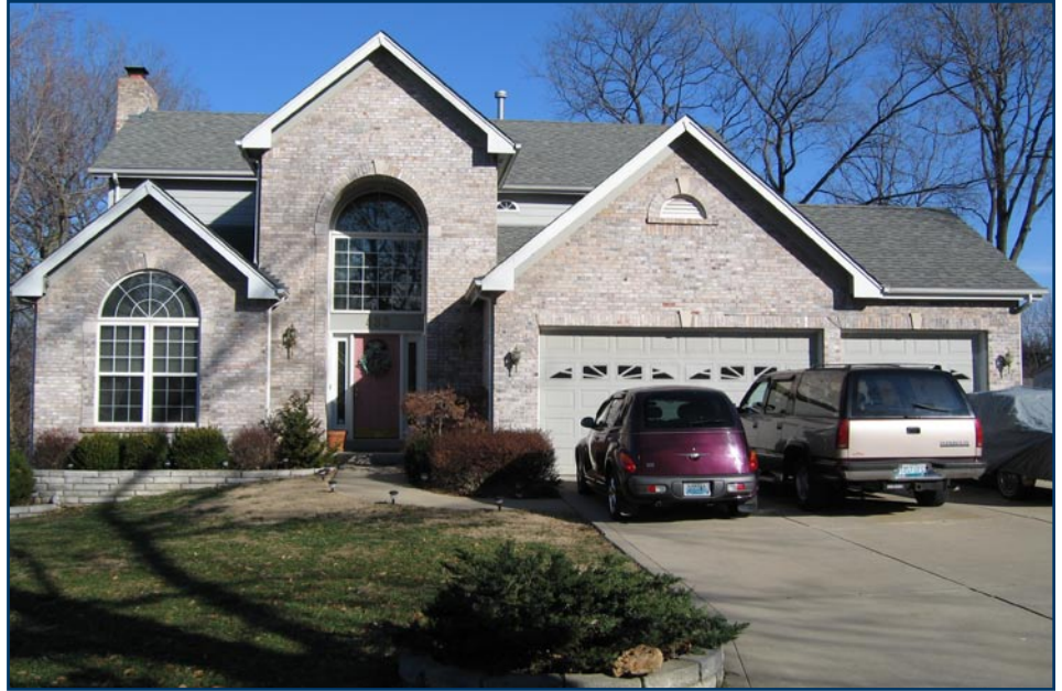
A Sunset Hills home condemned for blight.
